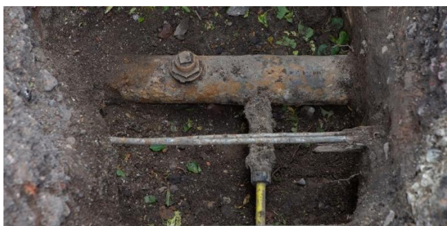
Figure 1: Yellow PE service tee off Steel mains
