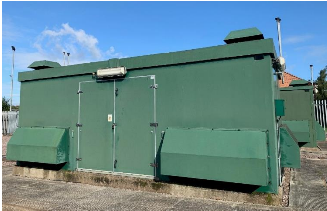
Figure 2: A typical GRP kiosk
